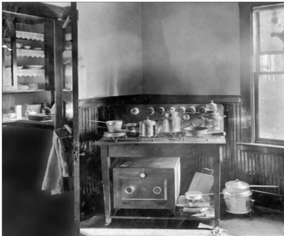
Electric Kitchen - Residence of H.W. Hillman - 1905
