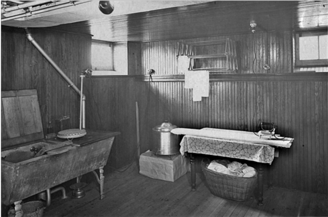
Immersion Heater, Wash Boiler and Electric Flat Iron, in Laundry of H.W. Hillman Residence 1905
