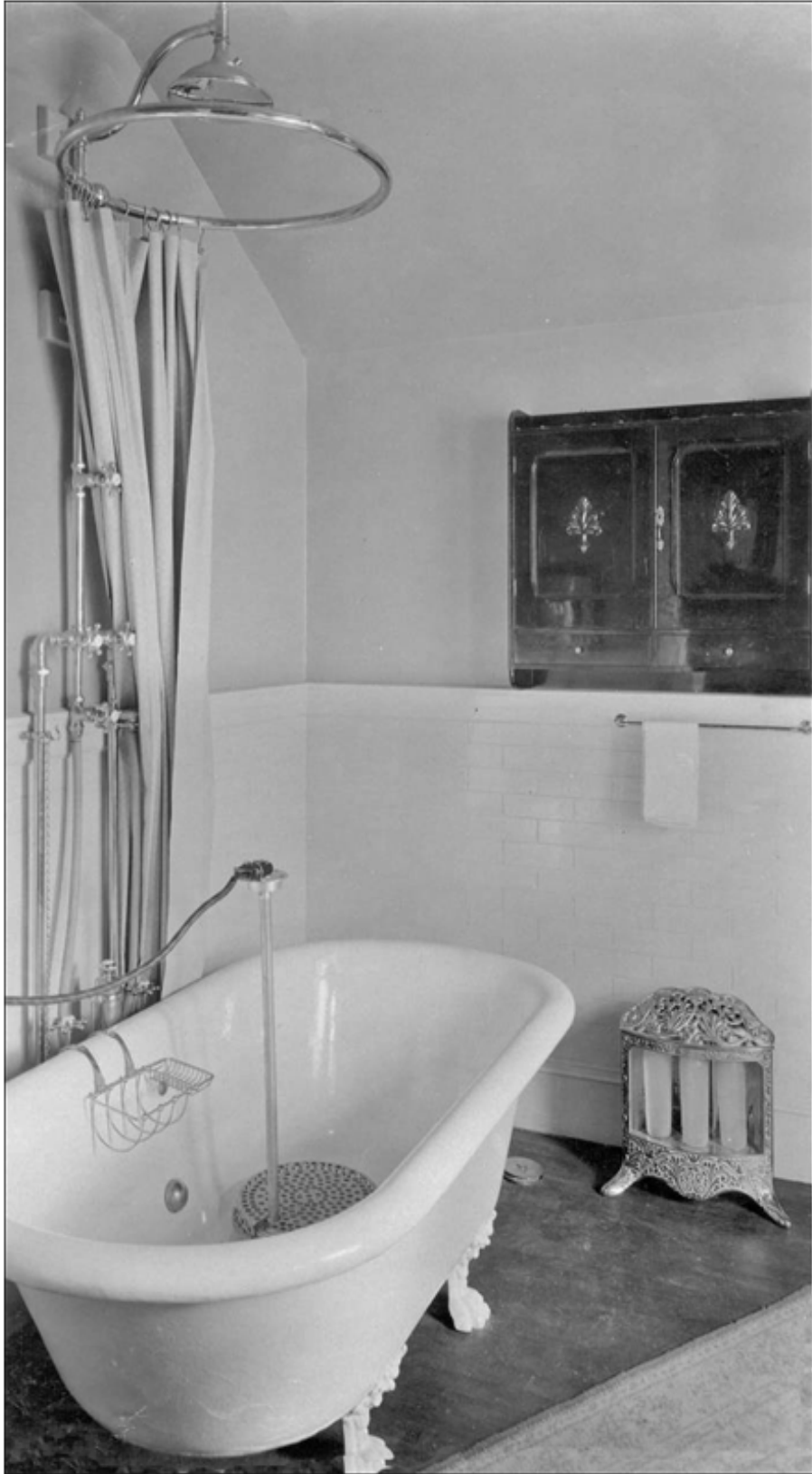
Bathroom showing Immersion Heater and Luminous Radiator - Home of W.H. Hillman - 1905
