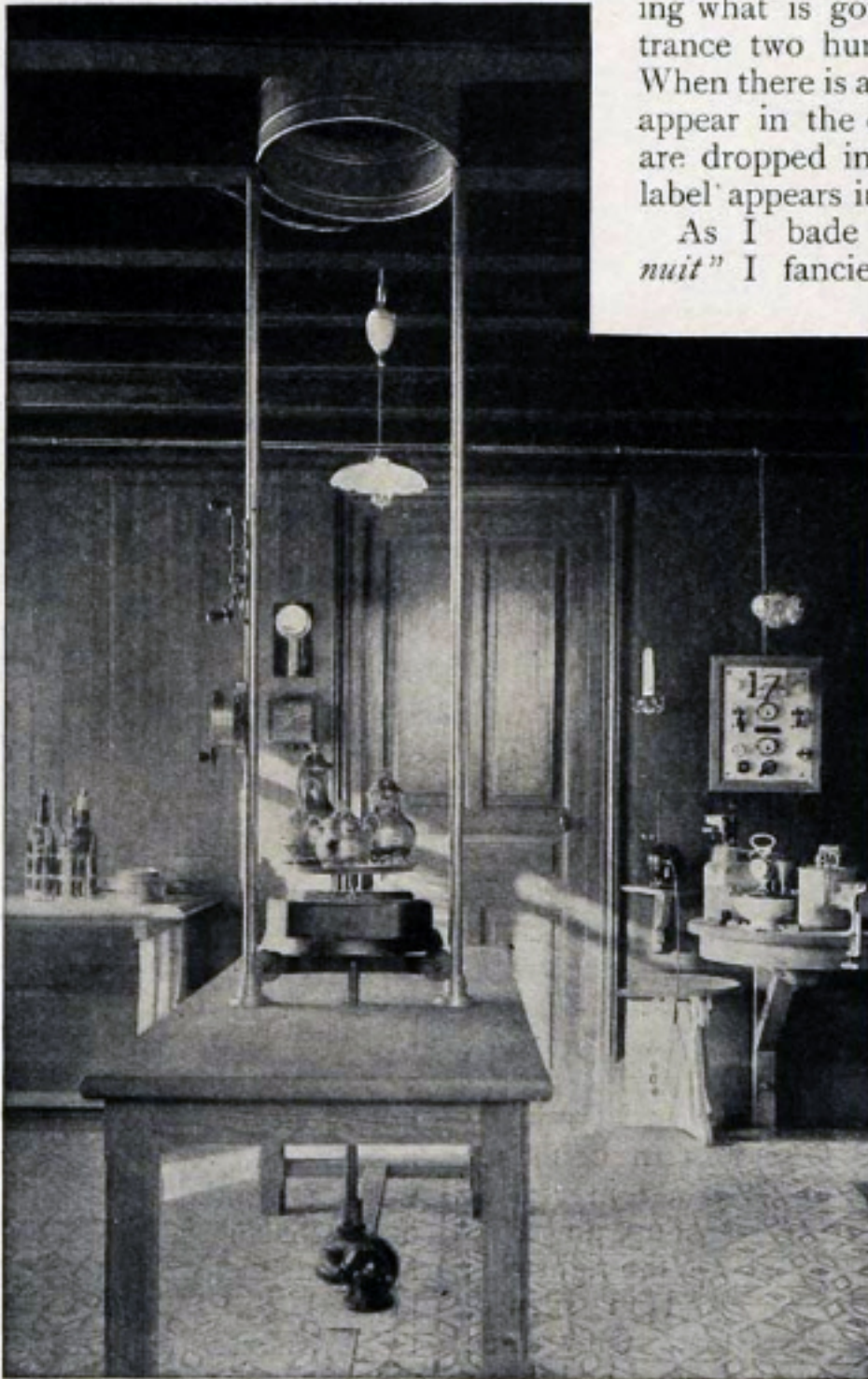
THE KITCHEN, WITH THE ELECTRIC LIFT TO CARRY THE DISHES TO THE DINING-ROOM, THE RANGE, WHICH RINGS A BELL WHEN THE JOINT IS SUFFICIENTLY COOKED, AND MANY OTHER REMARKABLE DEVICES.
