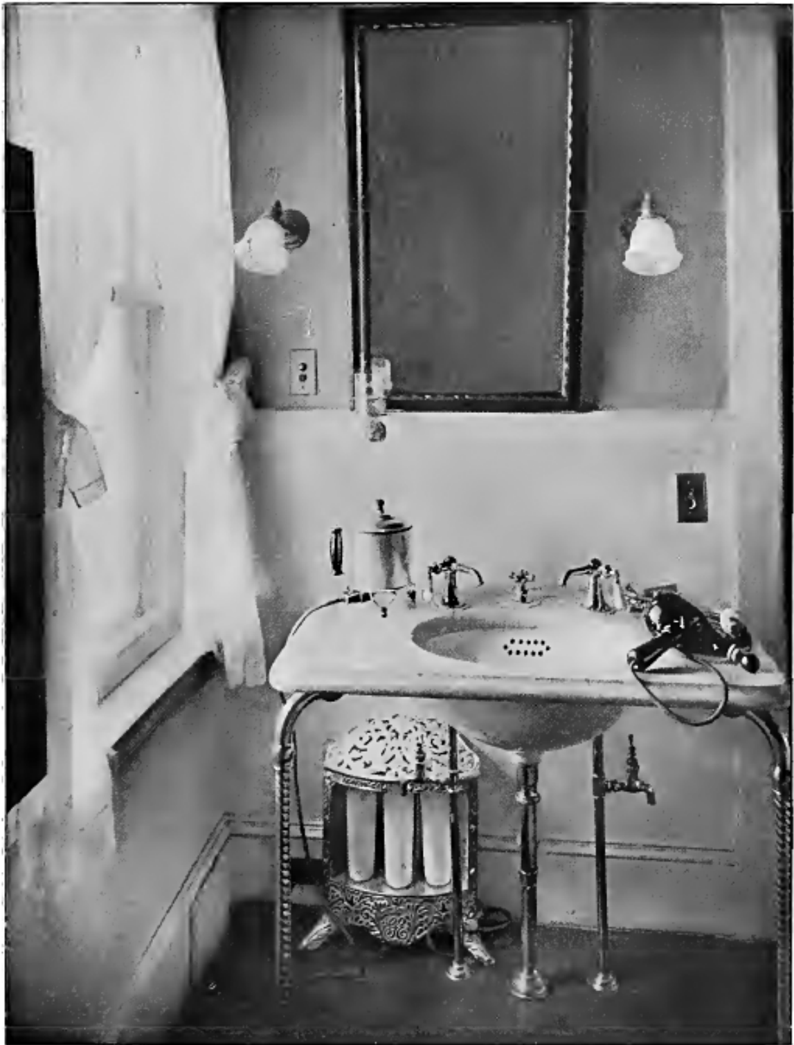
FIG. 7.—A PART OF THE BATH ROOM, WITH ELECTRIC RADIATOR, MASSAGE VIBRATOR AND WATER-HEATER FOR SHAVING
