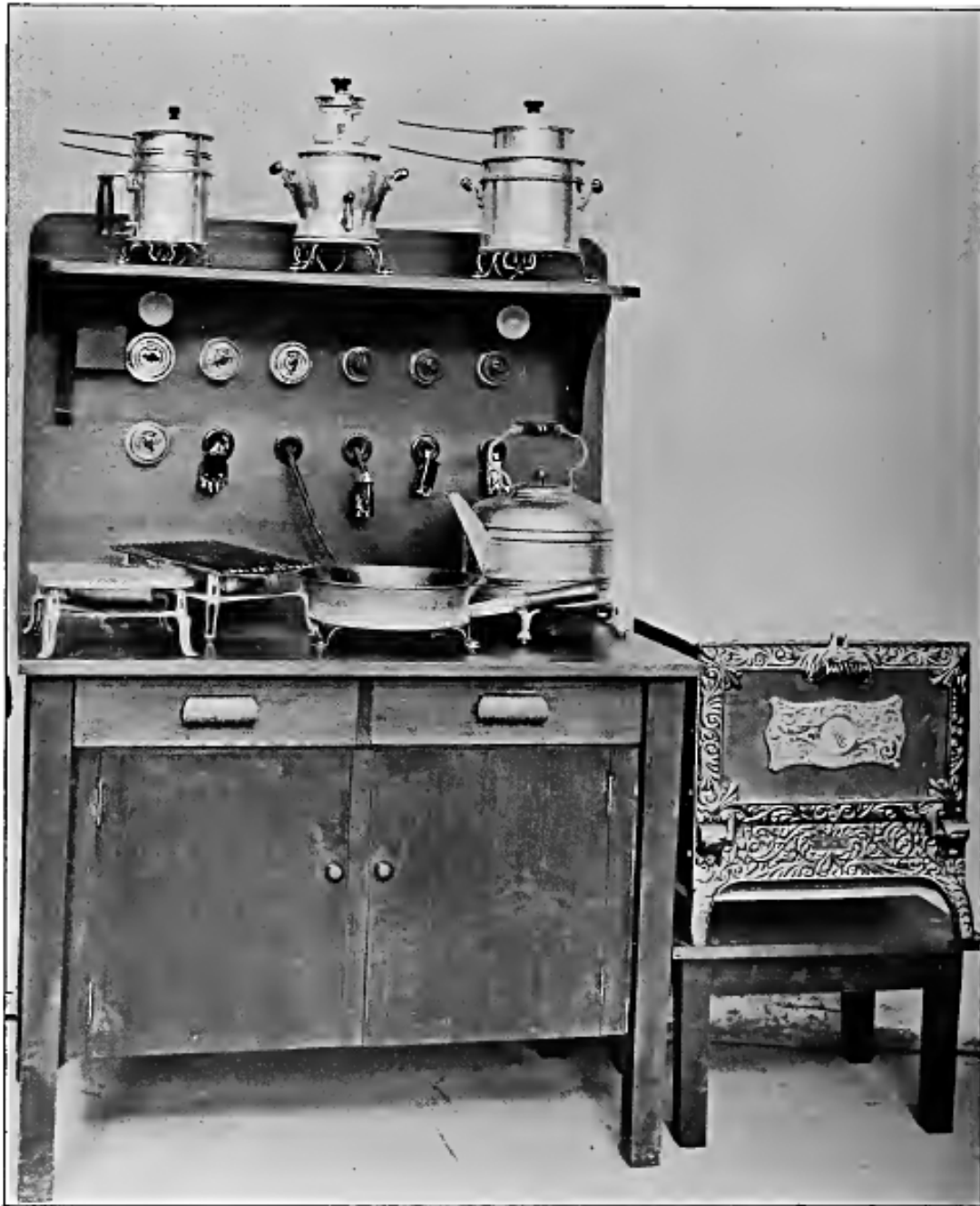
FIG. 8.—AN ELECTRIC COOKING AND BAKING TABLE, DESIGNED FOR A LARGER FAMILY THAN THE ONE IN FIG. 4
